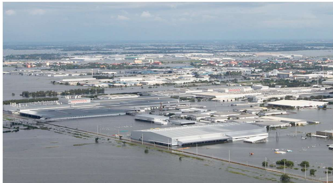
Flooding of Rojana Industrial Park, Ayutthaya, Thailand, October 2011.jpg http://en.wikipedia.org/wiki/File:Flooding_of_Rojana_Industrial_Park,_Ayutthaya,_Thailand,_October_2011.jpg
